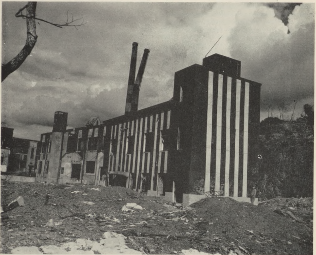
Photo 39. Photograph of one of the wings of the University hospital at Nagasaki, showing method of camouflage by applying black paint over portions of the yellow stucco finish. It was hoped to achieve an appearance of grayness at a distance to blend the building into the dark hills in the background.
